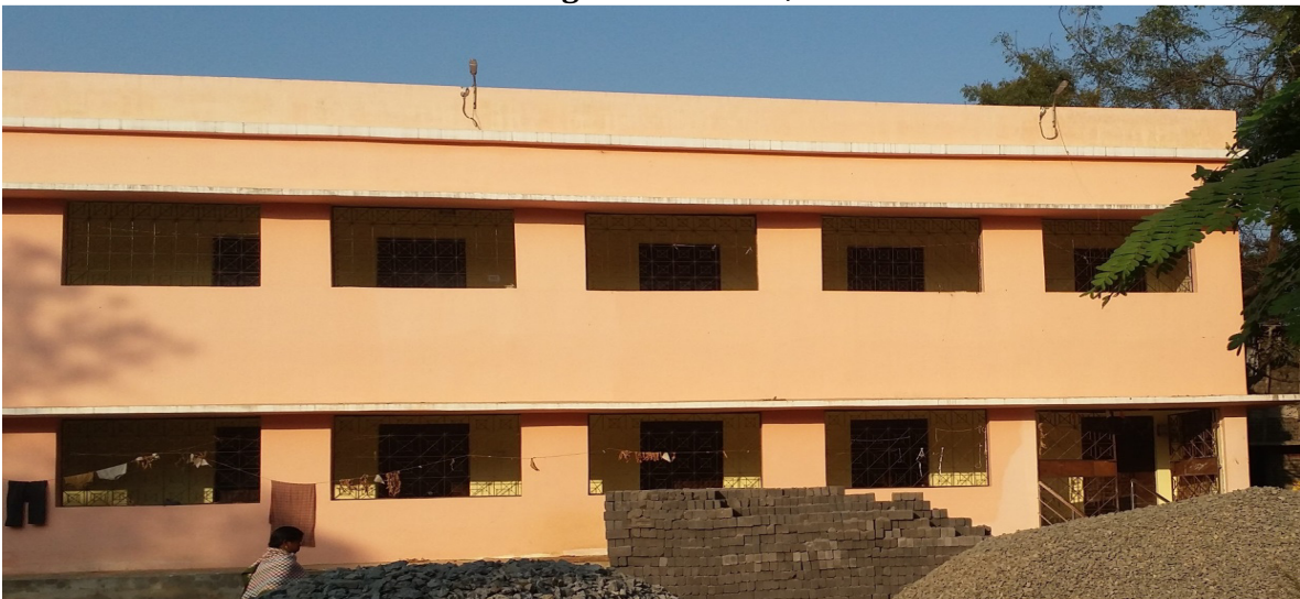
New Building of AWTC Unit-II,BARIPADA
